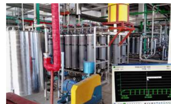
SMBR for alkali wastewater
